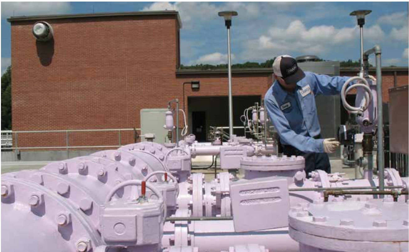
An Orange Water and Sewer Authority (OWASA) Operator checks the pumps at the Mason Farm Wastewater Treatment Plant in Orange County, NC. The plant delivers reclaimed water, or clean water repurposed from wastewater, to the UNC-Chapel Hill Campus, where it is used for purposes such as chilled water, landscaping irrigation, and more. Credit: Ed Kerwin
